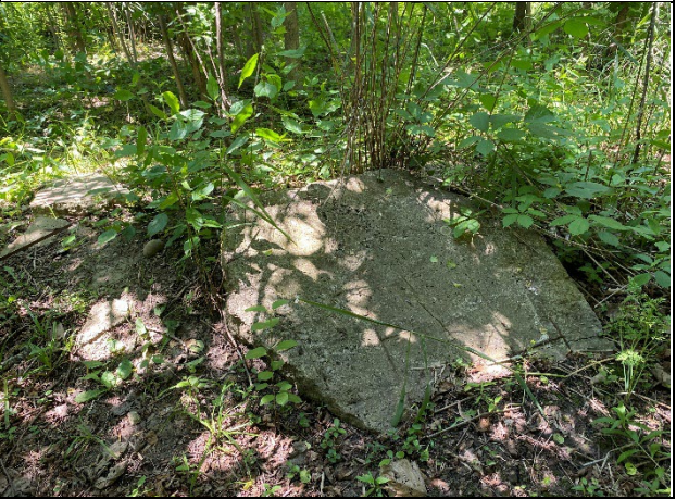
16. Large concrete slabs, attractive to snakes.
