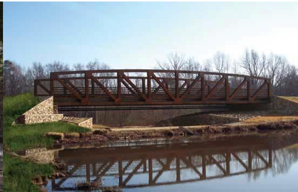
Pre-fabricated Steel Bridge
