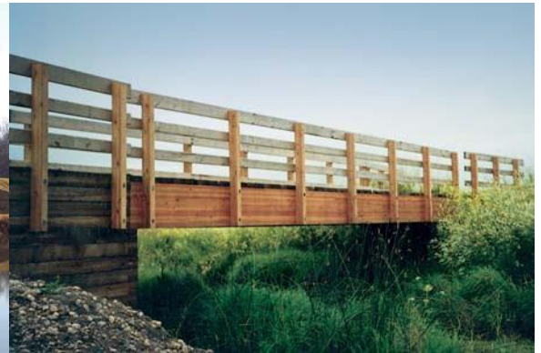
Pre-fabricated Timber Bridge
