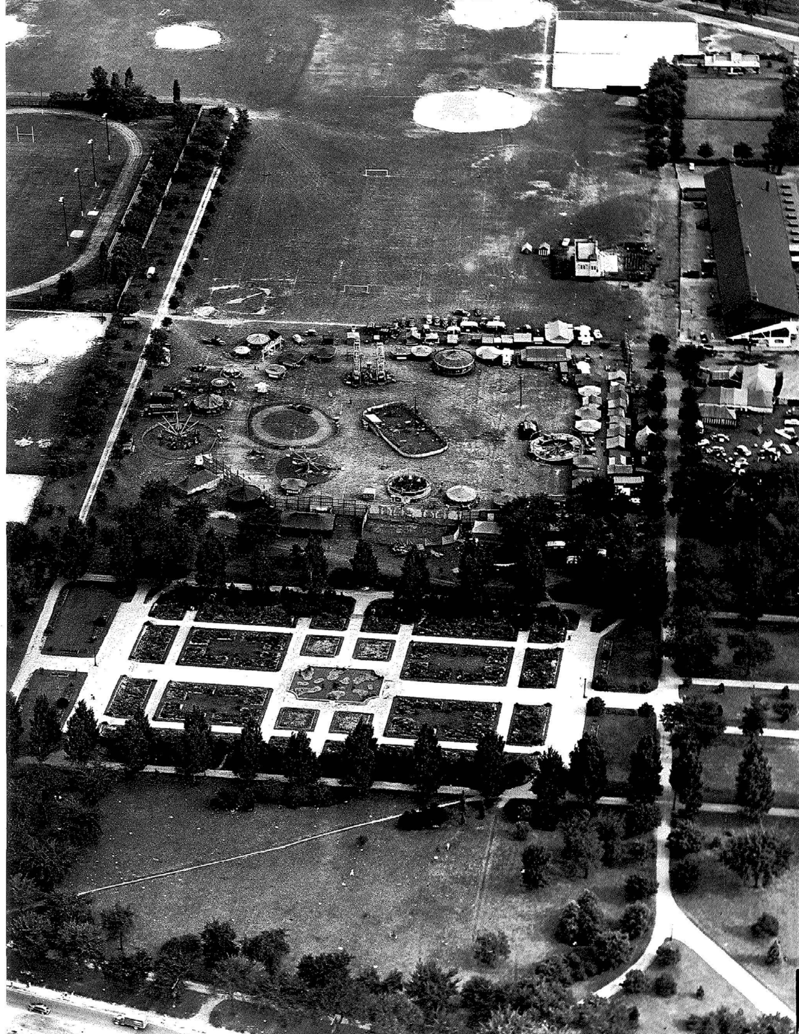
Figure 1-11: Aerial photo of Jackson Park (c. 1945)
