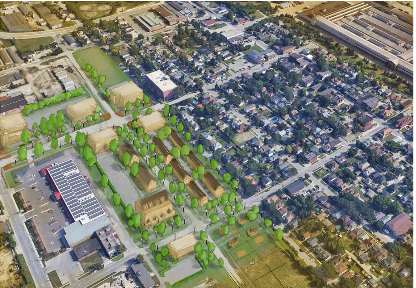
ABOVE: Concept highlights redevelopment opportunities for vacant industrial land between Walker Road and St. Luke Road, providing a gateway into Ford City where new roads physically link the Walkerville and Ford City neighbourhoods.
