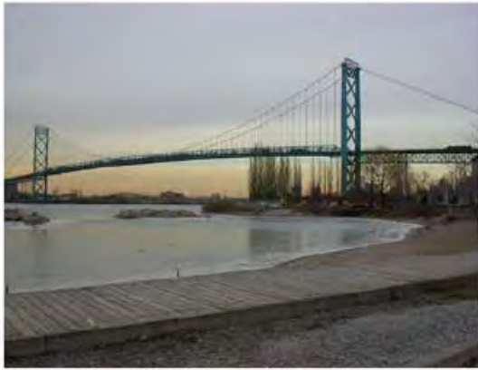
McKee Park on the Detroit River looking north towards the Ambassador Bridge
