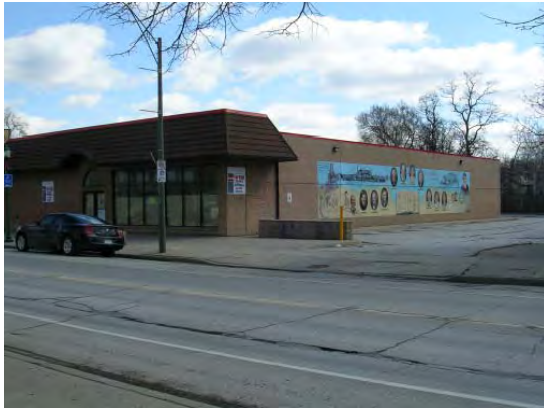
Vacant Store/Parking Lot at 3229 and 3235 Sandwich Street
