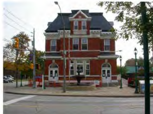
3201 Sandwich Street (Post Office)
