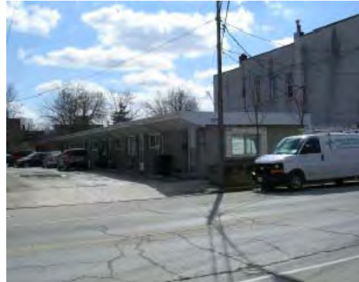
Former motel at 3173 Sandwich Street
