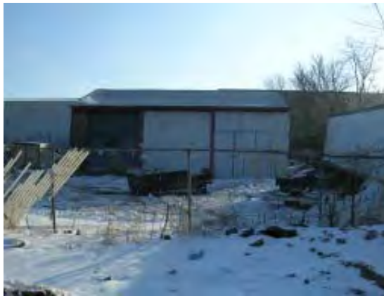
Derelict industrial building on Russell Street
