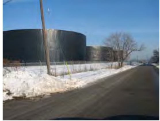
Fuel Storage Facility on Russell Street
