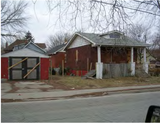
Boarded up houses on Edison Street
