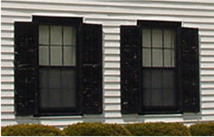
Windows and shutters on the MacGregor-Cowan House.
