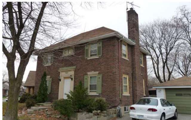
395 Rosedale Avenue. Note the Georgian Revival elements and sensitivity to the streetscape.
