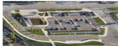
6. SEGMENT 7: AT GLENGARRY AVENUE (RTB SITE)
