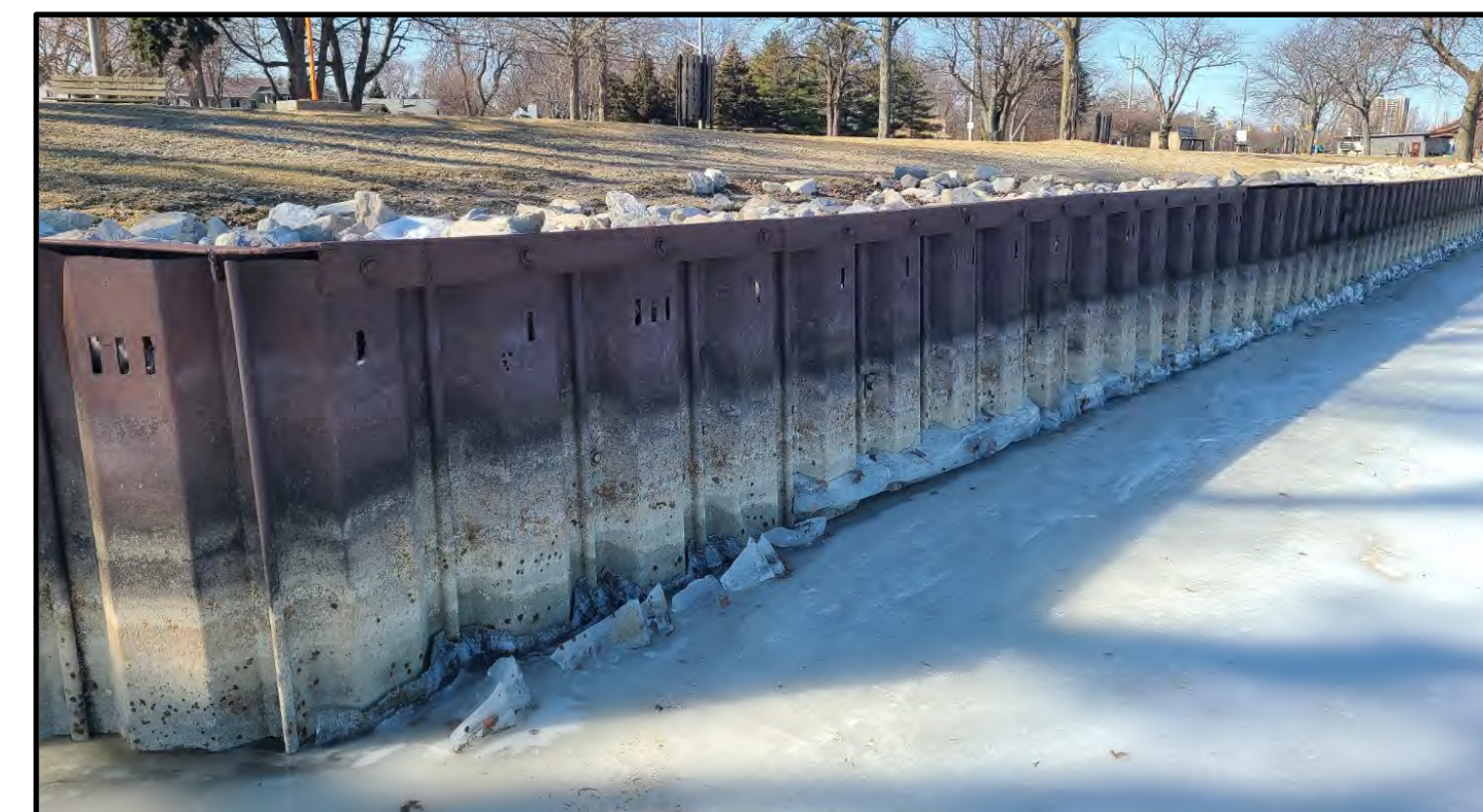
STEEL SHEET PILE SHOREWALL (SSP)
