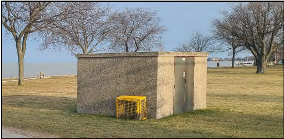
EXISTING STORAGE SHED (LESS THAN 40 YEARS OLD)
